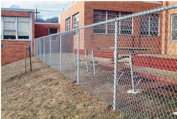
Galvanized Chainlink Fence
